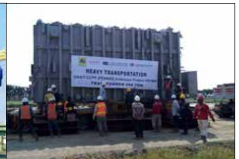
TRANSFORMER Transportation (LxWxH @ 11.8X4.4X5.5 M/288 TON)
